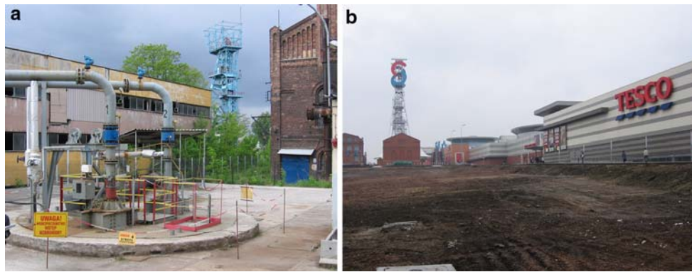
Fig. 8 Examples of abandoned mine sites in the Katowice area: (a) submersible pumps in the the abandoned (but still dewatered) Katowice mine, adjacent to the Spodek stadium and the proposed
